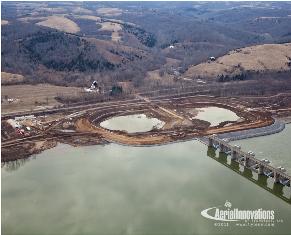
Meldahl construction February 2011
