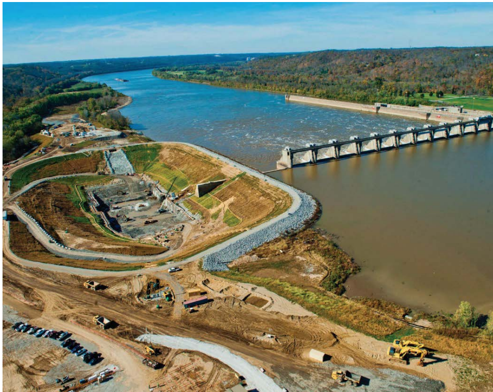
Meldahl construction October 2011
