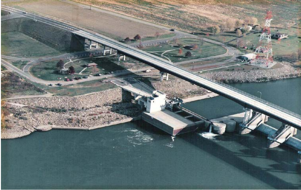
Greenup Hydroelectric Plant
