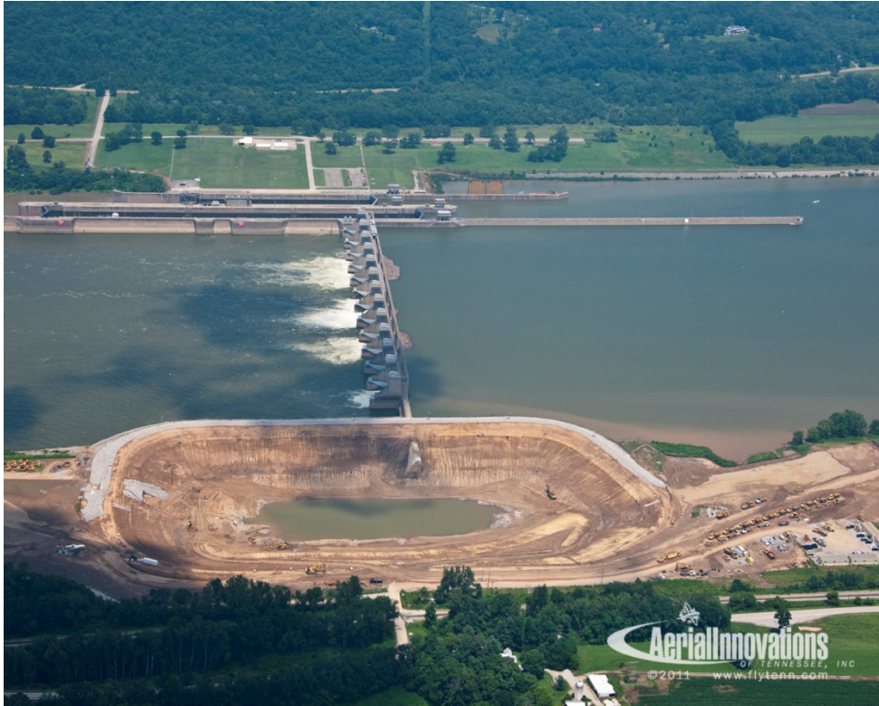
Meldahl construction July 2011
